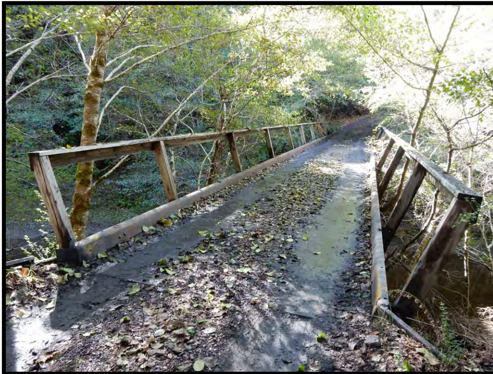
Figure 12: Photo Point #17- Bridge to Reist Ranch /Hollow Tree Creek
