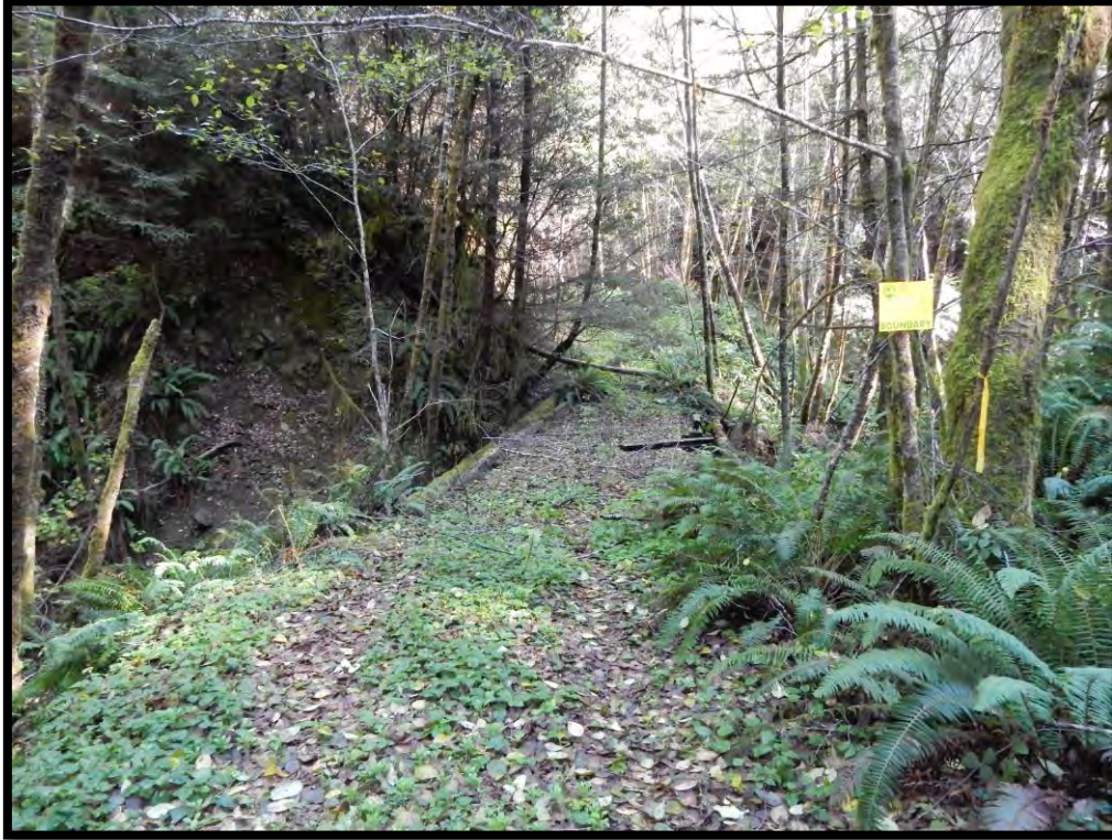
Figure 3: Photo Pint #3- Usal Creek Bridge on road to Julius Creek, Bridge #16.
