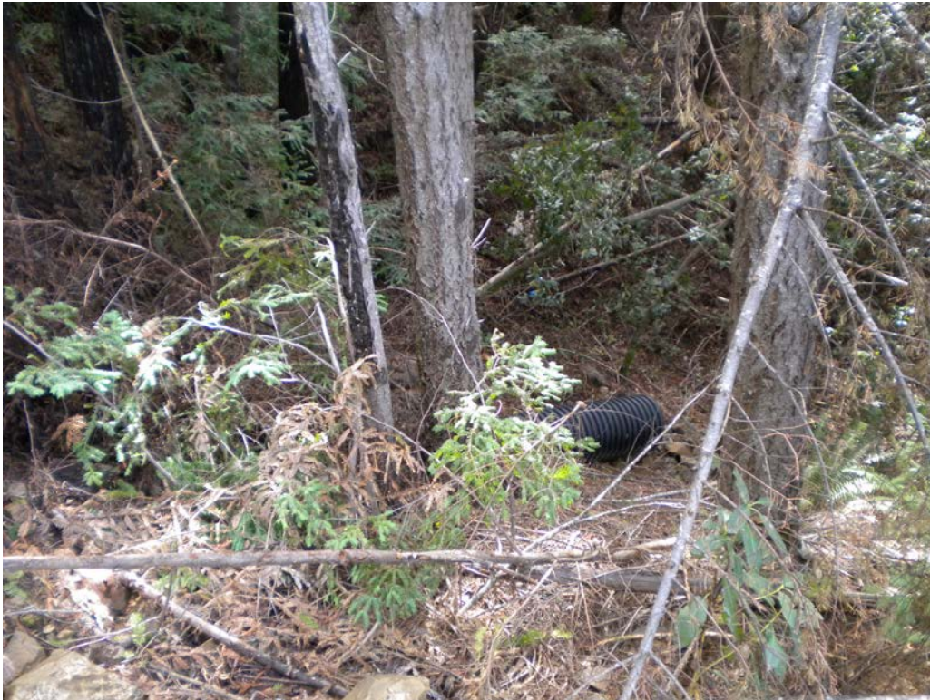
2014 Photo Point 3. WRP Road, THP related culver replacement.
