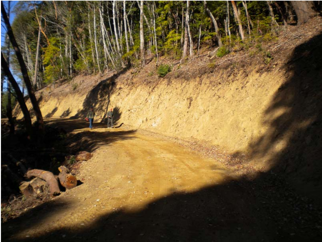
2013 Photo Point 2. New road built by Mendocino Redwood Company.
