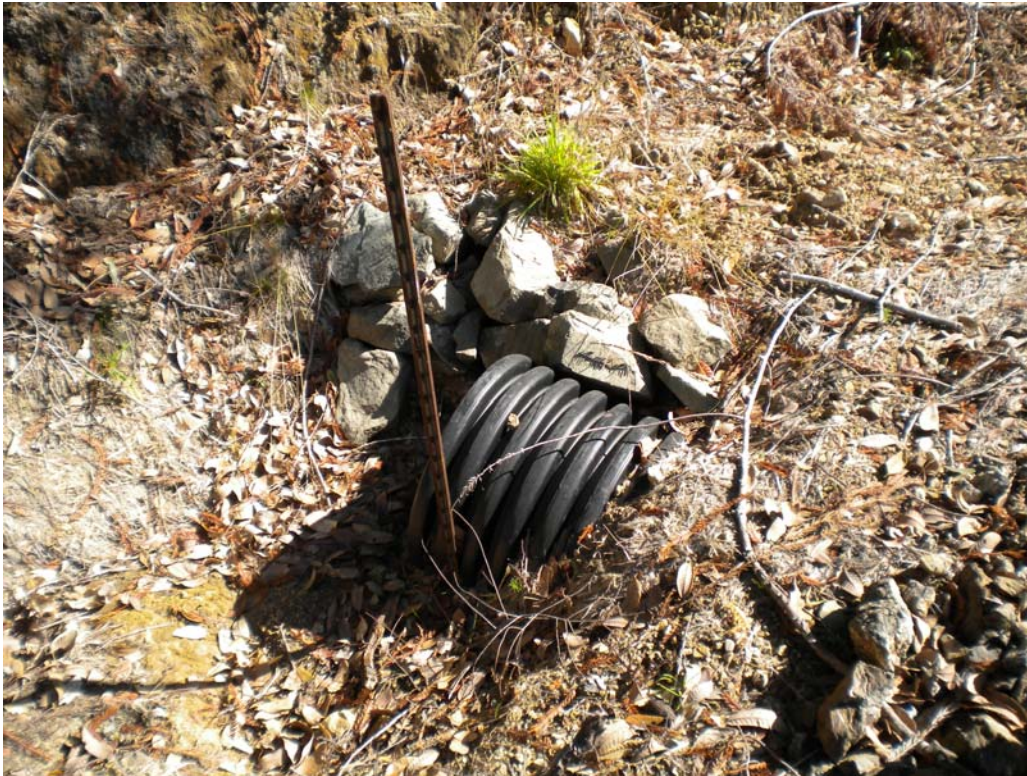
2013 Photo Point 6. M&M road culvert replacement, after first winter.
