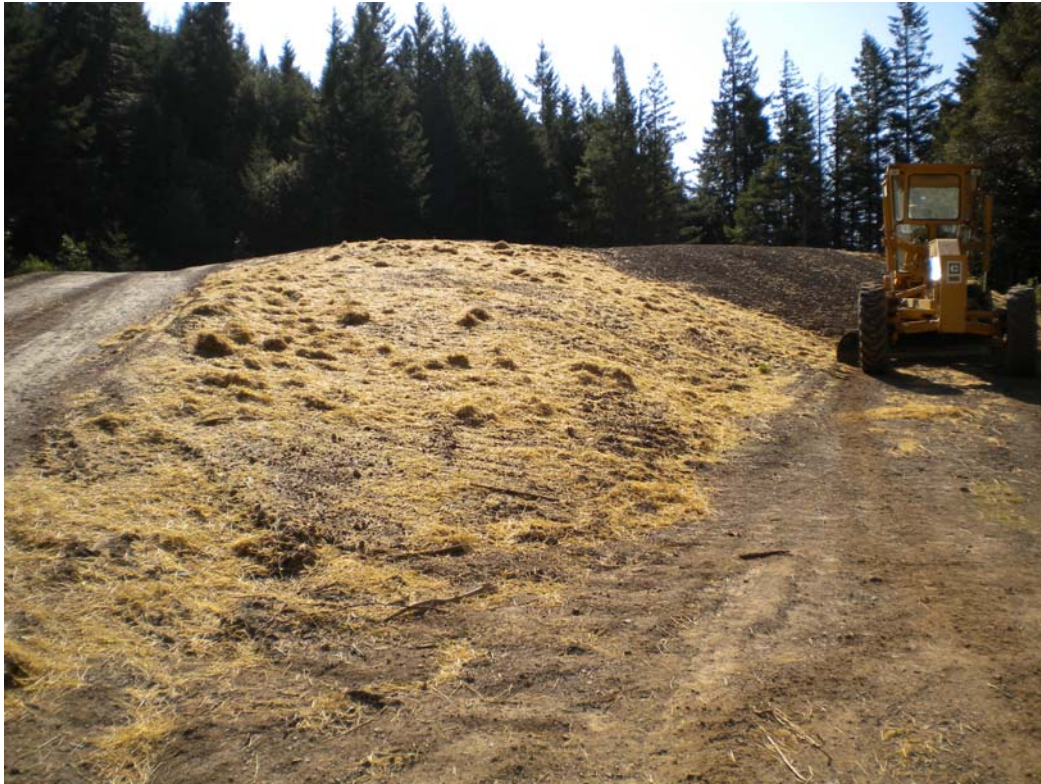
2013 Photo Point 3. Spoils from new road built by MRC; placed on Usal Forest landing.
