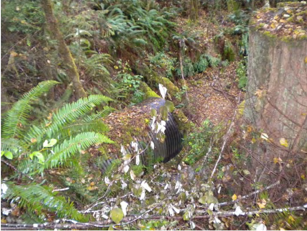
2012 Photo Point 3. Elevated culvert on M&M Road.
