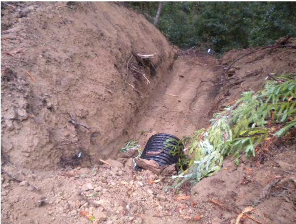
2012 Photo Point 2. M&M Road, new ditch relief culvert.
